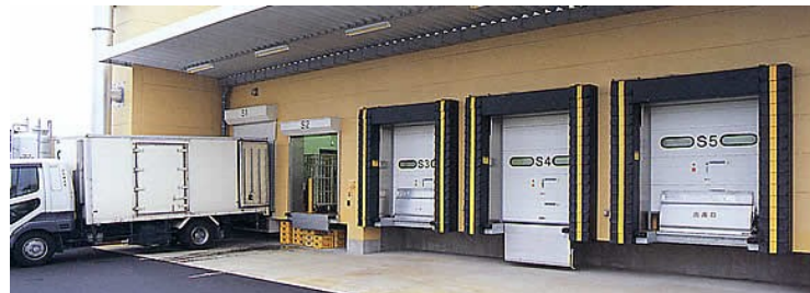
Loading Dock Shelter's Curtain
