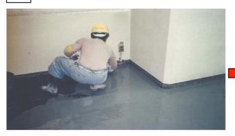
Apply Short Filler equally for the 1st time with the amount as much as the setting bed should not be appeared. Apply for the 2nd time after the 1st time completely dried (After about 30-60 min at a set temperature) which is as much as the way lets constructor walk on with clean shoes.
