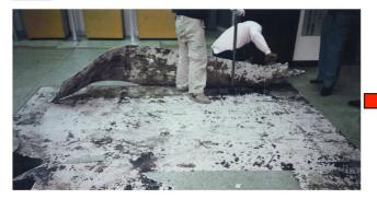
Remove off the existing sheet and check the condition of the setting bed surface
