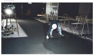
Smoothly toweling by steel trowel after About 10-20 min at a set temperature.
