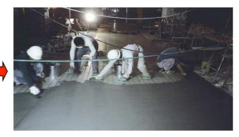
Apply Short Filler twice. Apply the amount as much as the setting bed should not be appeared. (About 0.5thickness)
