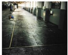
Vacuum dust after removing off the floated and deteriorated portion
