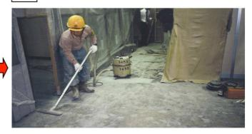
Sprinkle HANEDA Sealer undiluted solution sufficiently, clean it off with a deck brush, scrape it off with a squeegee, and dry.
