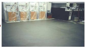
Smoothly toweling by steel trowel after About 10-20 min at a set temperature.
