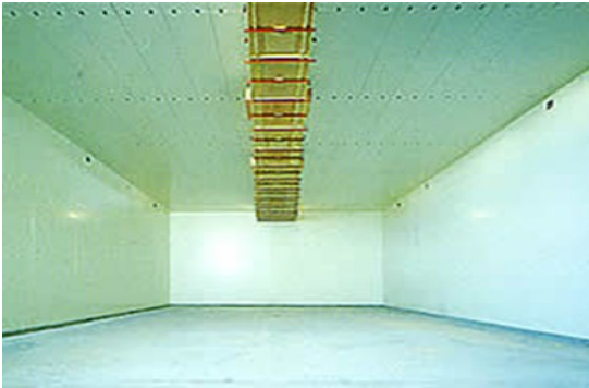
▲ Large prefabric freezer with SOGO's airconditioner units delivered and constructed at one time
